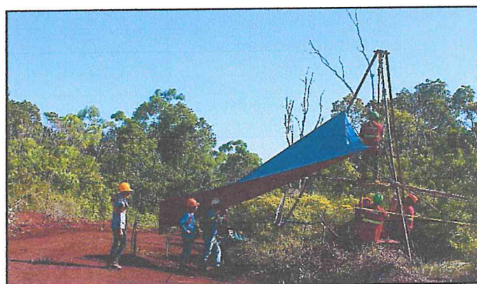
Core drilling at Hole ID R8+50N+100E.
