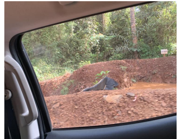
Photo 9. Silt traps along the drainage canal
