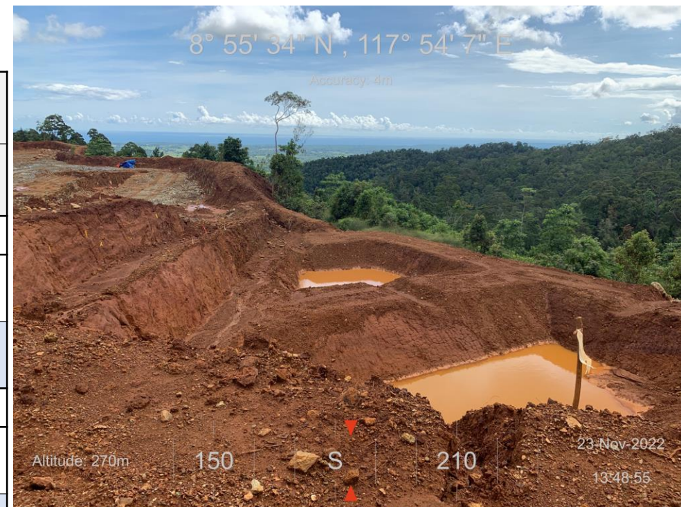
Photo 7. Check dams along the perimeter of the active mining area.
