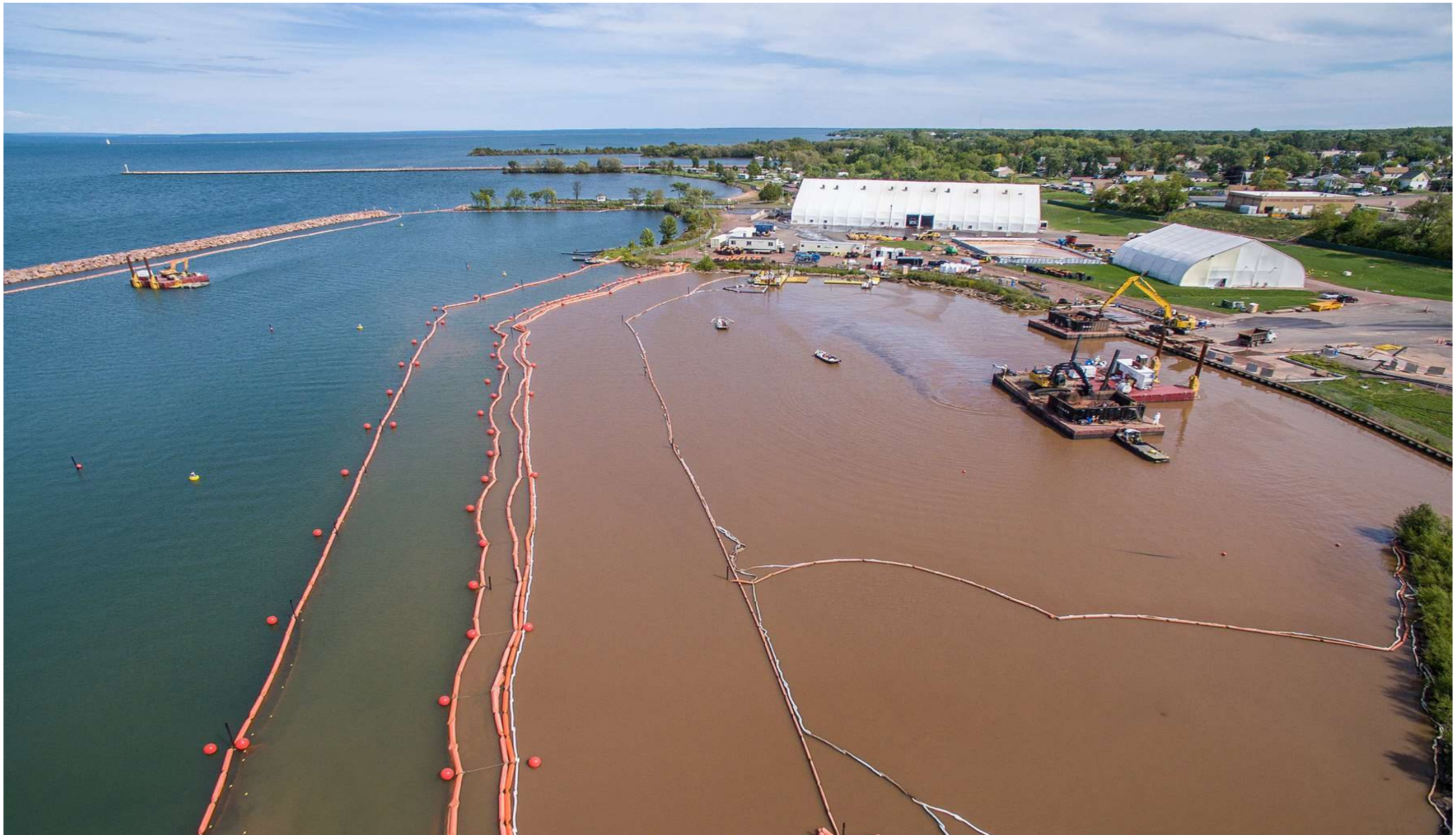
Figure 3_Sample of Silt Curtain installation to contain disturbed water from polluting other parts of Mindoro Strait that can damage or destroy marine habitat.
