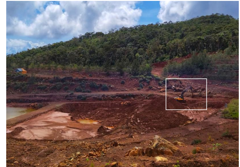
Photo 16 – 17. Ongoing desilting activity at Block B SP No. 1 (top) and SP No. 2 (bottom) during the time of monitoring.
