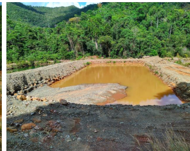
Photos 11 – 12. Desilted compartments - second compartment (left) and first compartment (right) – of Old Communal Dam SP during the 3 rd Quarter.
