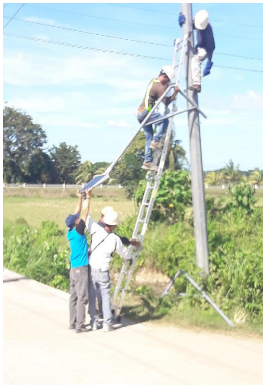
Plate 5.23. Installation of Solar Powered Street light along Sityo Casoy, Central, San Jose, Occidental Mindoro
