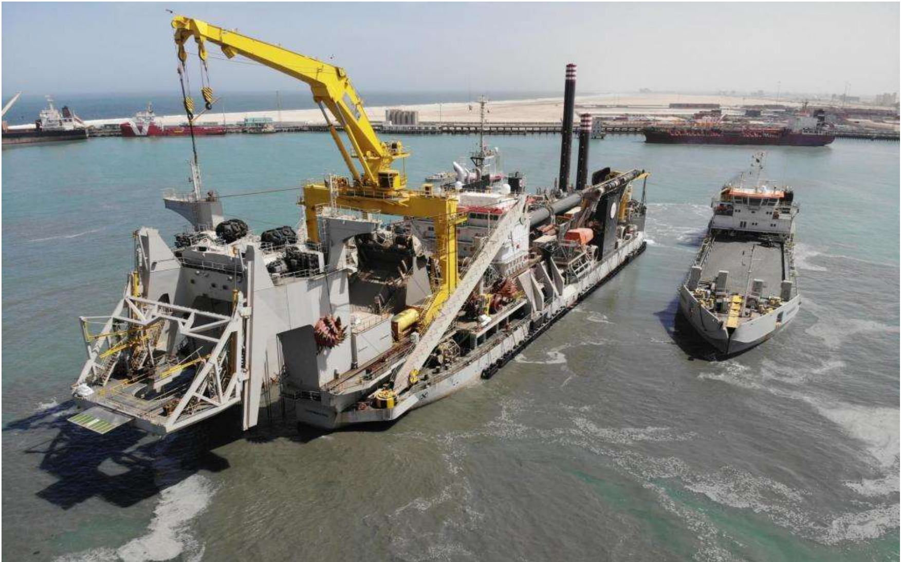
Figure 3_Cutter Suction Dredger and barge.
