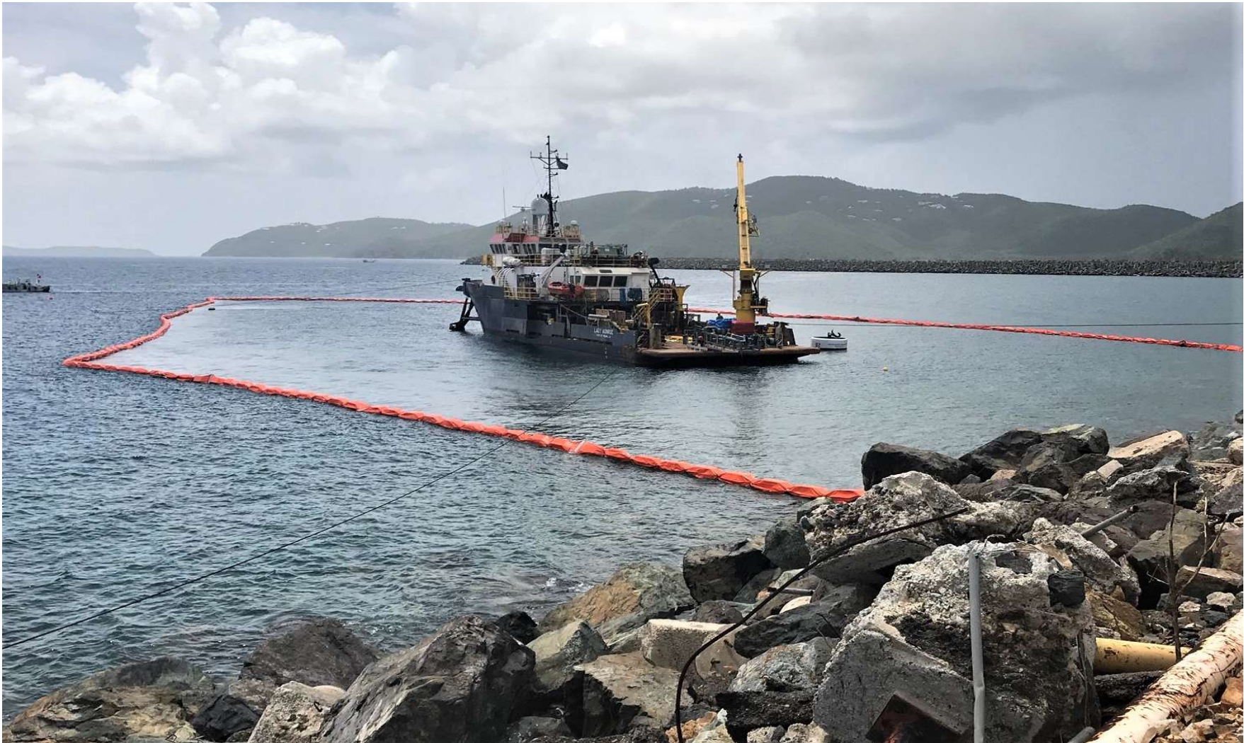
Figure 4_Sample of Silt Curtain installation to contain disturbed water from polluting other parts of Tablas Strait that can damage or destroy marine habitat.
