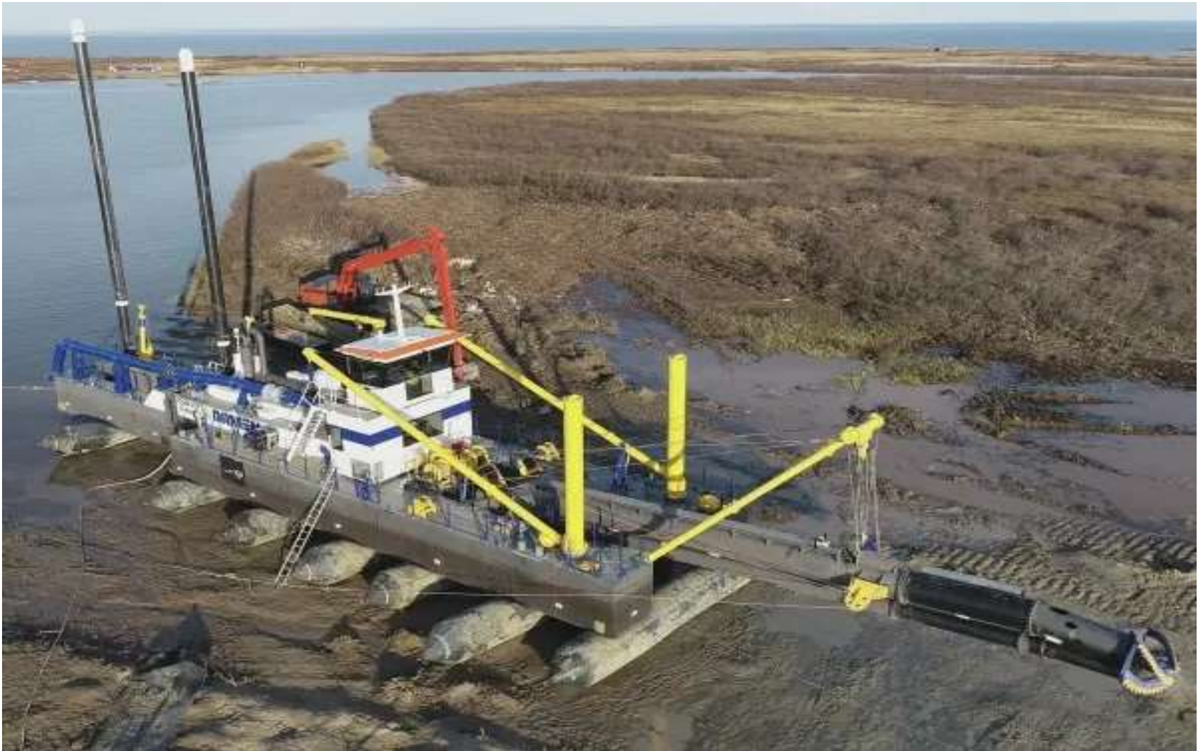
Figure 2_Cutter Suction Dredger – Damen CSD 250, showing 2 spuds to position the dredger steadily.
