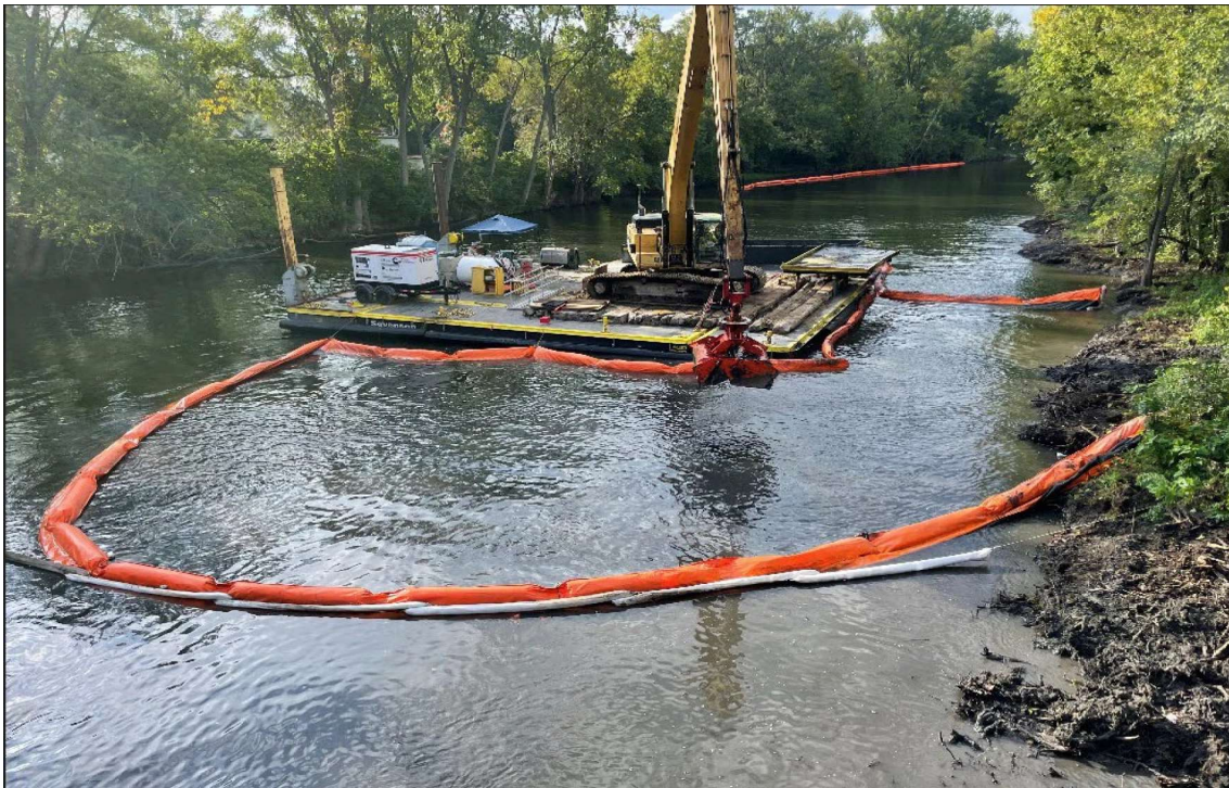
Plate 7 _River Dredging using barge with long-arm excavator to remove the sediment with silt curtain to prevent turbidity from spreading at Allied Paper-Portage Creek-Kalamazoo River. Source: Michigan Radio.org – US EPA
