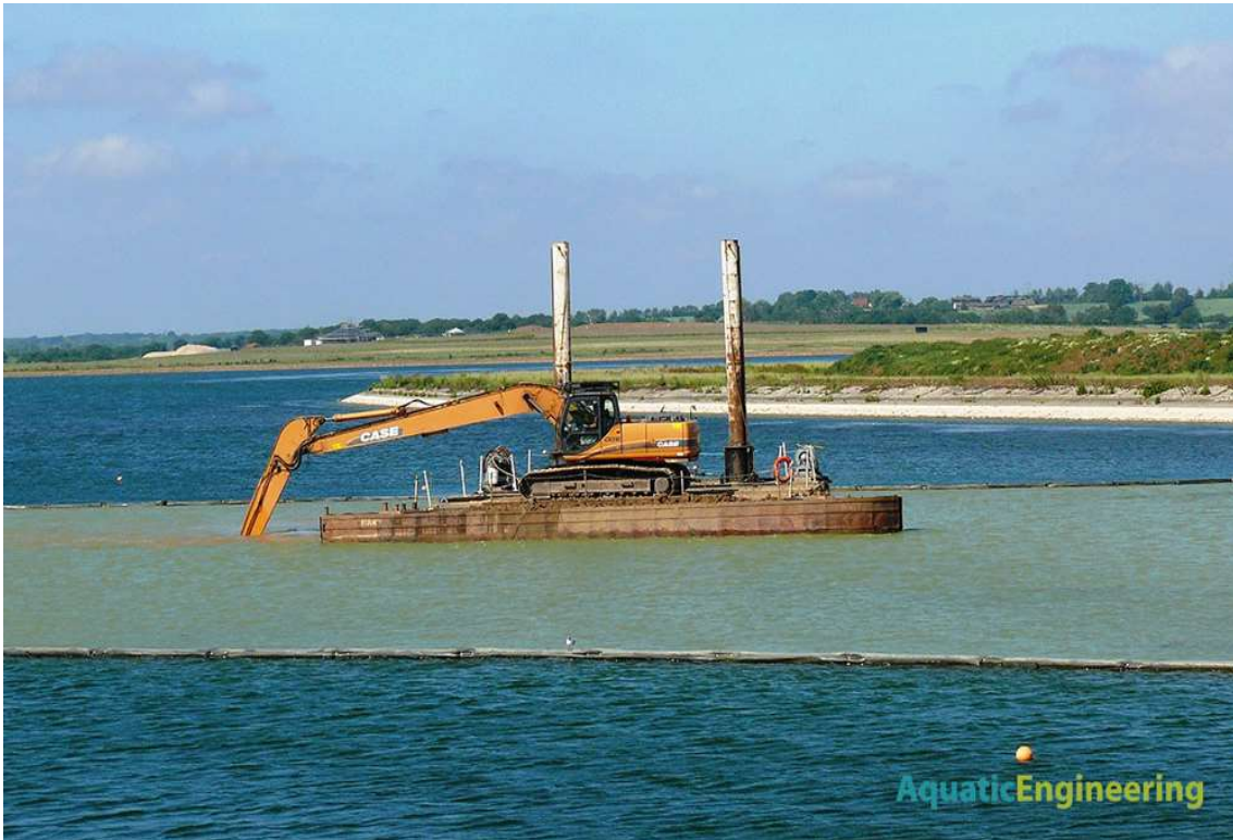
Plate 6 _Typical Silt Curtain Installation. Source: Aquatic Engineering https://aquaticengineering.co.uk/difference-silt-curtain-and-turbidity-barriers/
