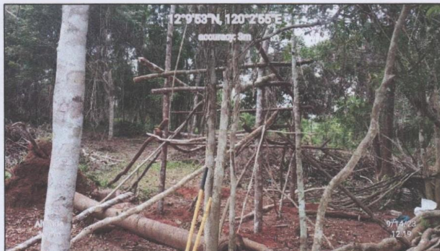
Figure 3. Documentation of ongoing construction of house structure made of round timber purposely for their generator
