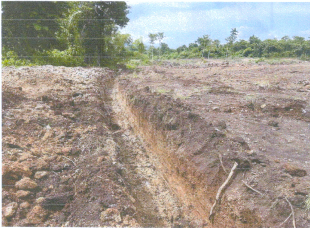
Photo 3. Temporary drainage canal with a length of approximately 50 meters that has been constructed at the proposed project area.
