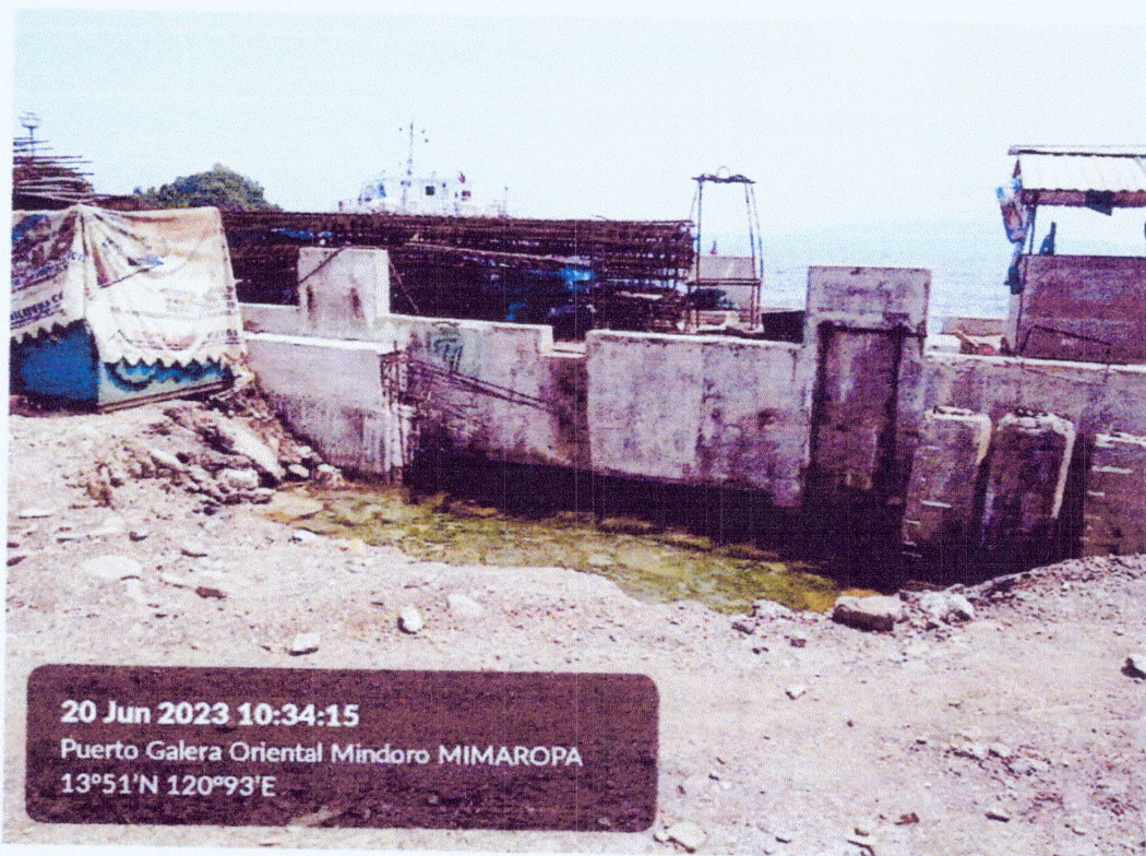
Photo 2. On-going construction of finger pier.
