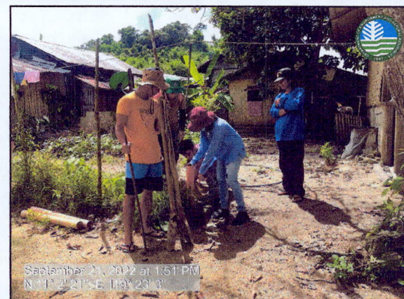
Photos during layout and the placing pvc pipes marker on the delineated 40-meter easement zone.
