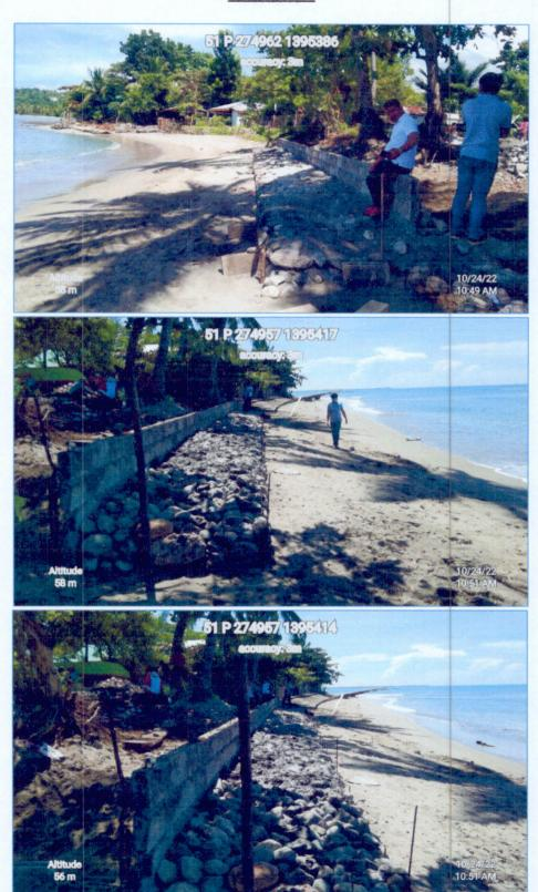
The on-going construction of concrete seawall (length = 20 meters; width = 2.5 meters; height = 1.5 meters) made from various materials such as rocks, cements, steel bars, hollow blocks, sand and gravel.
