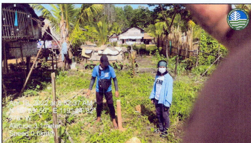
Placing pvc pipe marker of the delineated 40-meter easement/buffer zone within mangrove area.
