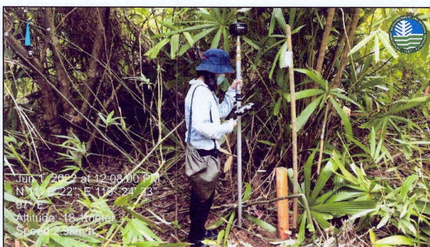
Locating and placing of the pvc pipe marker for the 40-meter easement/buffer zone.
