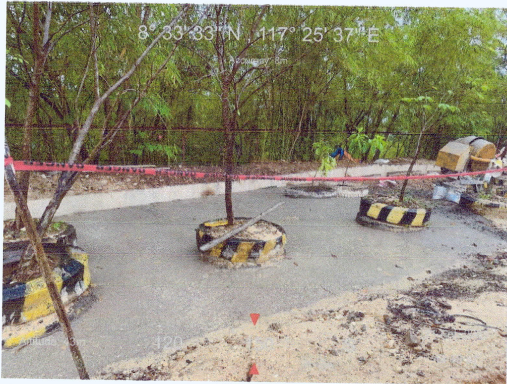
Continuous road concreting inside the plant site
