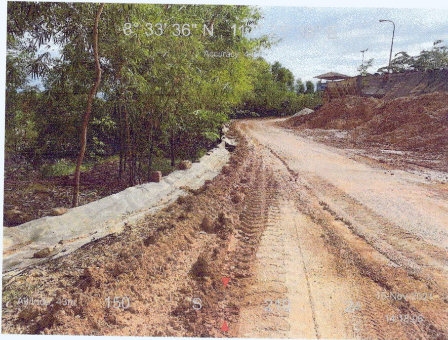
Accumulated silt on the concrete road near the limestone feed stockpile was again observed. For Immediate removal.
