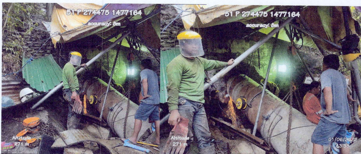
On-going repair of the damage Pipeline at the back of Power House
