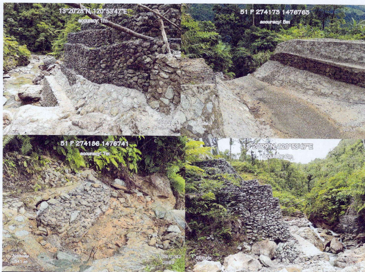
Newly construction gabions along creeks for river bank protection
