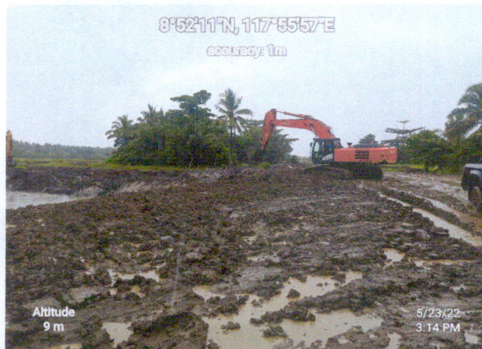
Pictures above showing the construction of siltation pond
