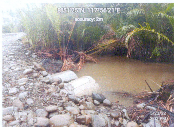
Pictures showing the installation of culvert to protect the naturally flow of water
