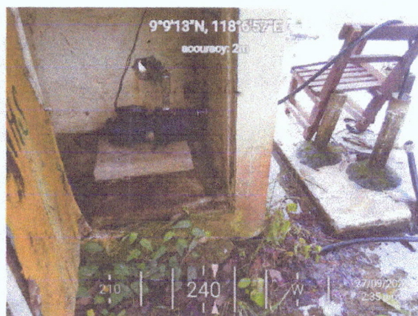
Electric-motor water-pump used by Doris Martinez National High School in withdrawing natural ground-water (deep well)
