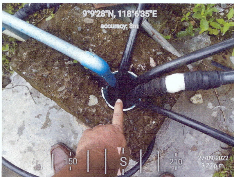
LGU Abo-abo Brgy. Hall : natural ground-water (deep well) : approximately 40 meter deep.
