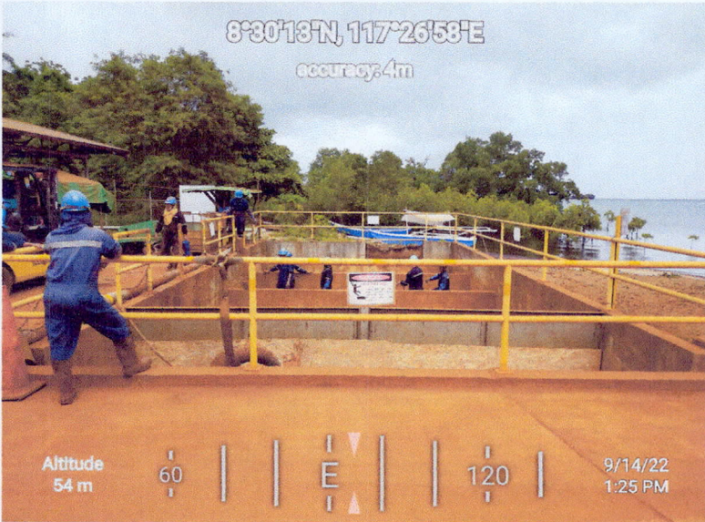
Concrete Siltation Pond
