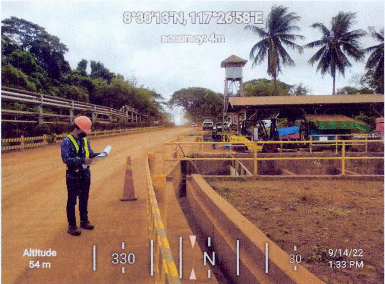
Drainage areas pass through to concrete siltation pond
