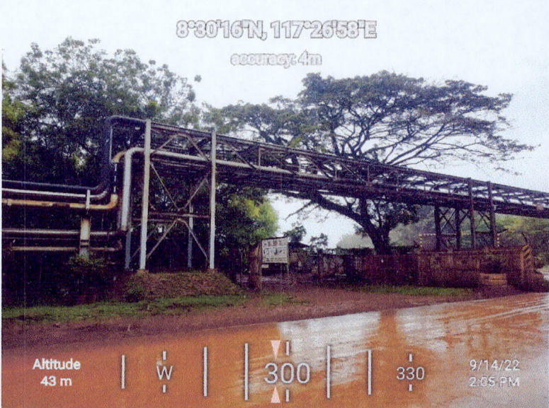
Steel posts with built-in metal pipe lines
