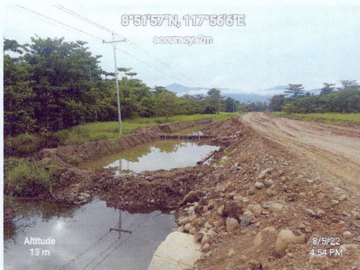
Pictures showing the silt trap with installed geo textile located along dikes near the hauled road of Ipilan Nickel Corporation (INC)
