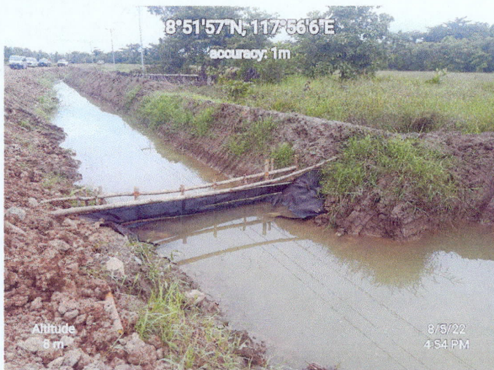
Pictures showing the silt trap with installed geo textile located along dikes near the hauled road of Ipilan Nickel Corporation (INC)
