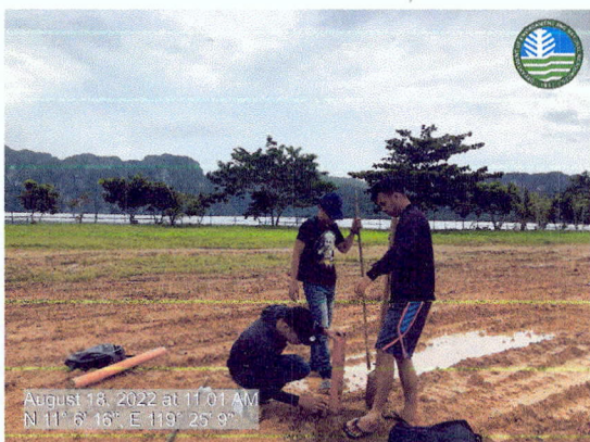
Photo showing the placing pvc pipes marker on the ground.
