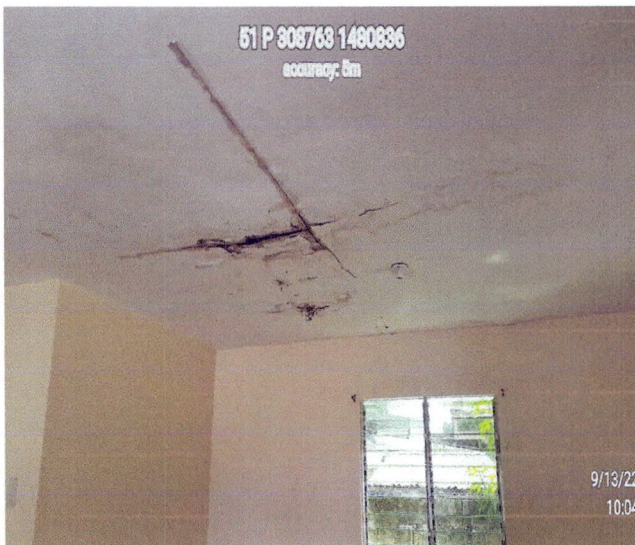
Leaking roof and damaged ceiling of information center.
