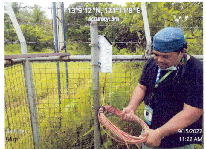
Maintenance and Monitoring of Ground Water Level Monitoring Station instrument at Mindoro State University Compound, Victoria, Oriental Mindoro last September 15, 2022.
