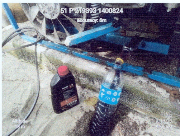
Figure B.3. Changing of oil of the compressor.
