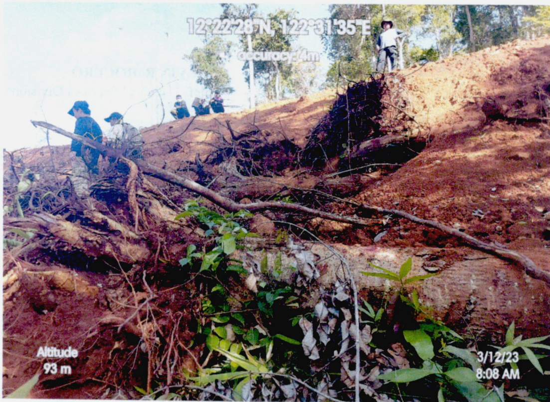
Uprooted trees dumped and filled with soil on a cliff beside the perimeter access road
