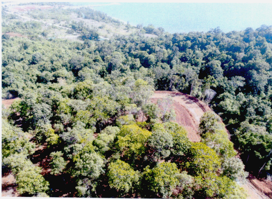
Aerial photos of the perimeter access road within the 20-hectare site of APMC
