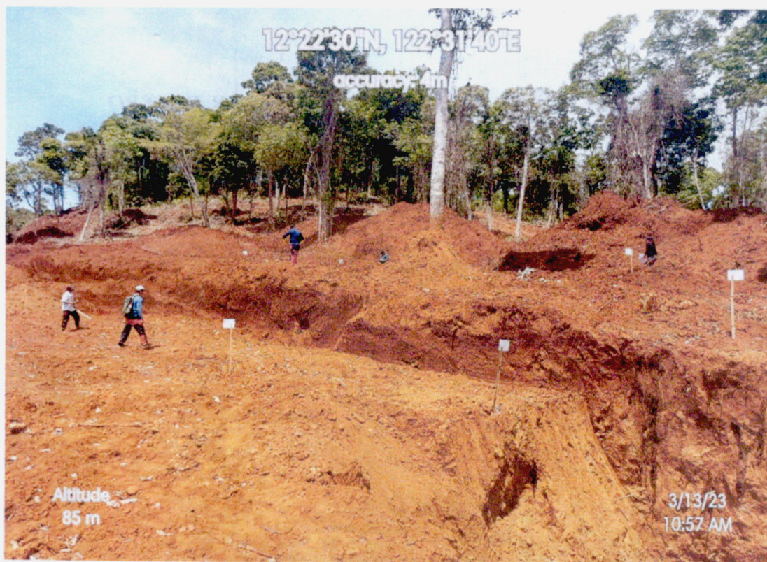
Staking and marking of missing trees
