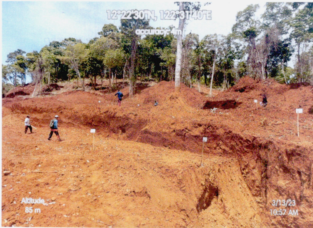
Staking and marking of missing trees
