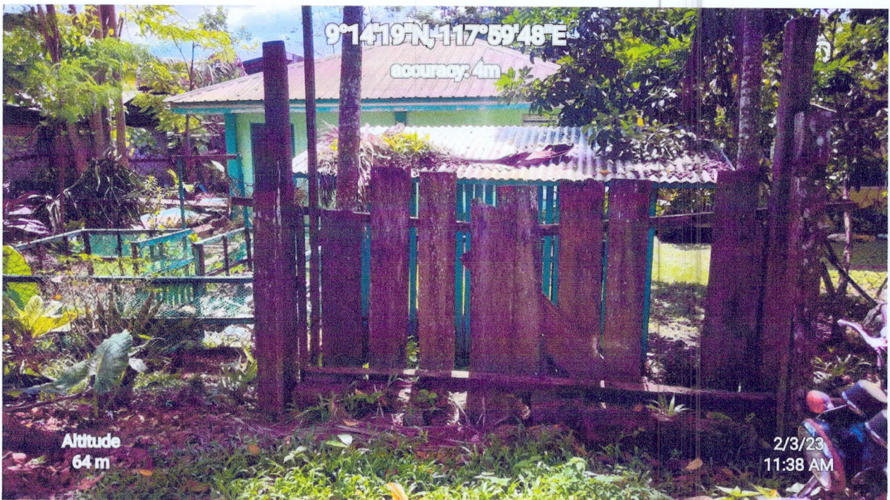
Geo-tagged pictures showing the rotten and broken fence of CENRO-Quezon, Palawan.
