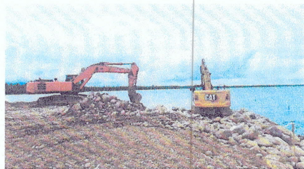
Picture Nos. 36 & 37: Left- Dumping of Armor rocks at the east portion of Phase 2; and Right – Placing the core and armor rocks (taken Aug. 4, 2022 PM)
