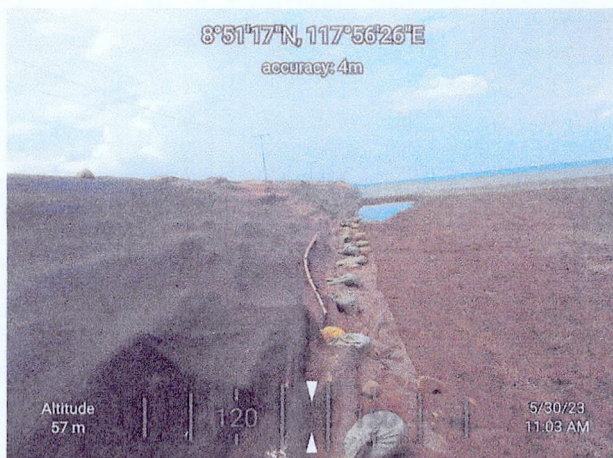
Installed silt fence to avoid erosion of backfilled materials
