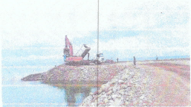
Picture Nos. 34 & 35: Left- Causeway's L-portion (Phase 2) measures 30m x 30m long as of August 4, 2022, while dumping activities continues (Right)
