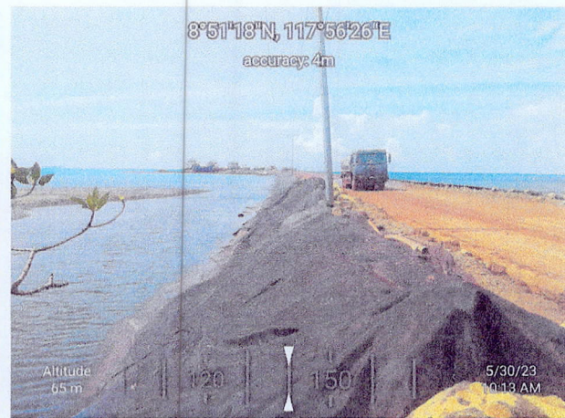
Installed silt fence to avoid erosion of backfilled materials
