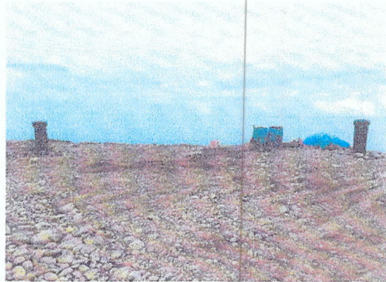
Picture Nos. 38 & 39: Left- L-shape of the causeway now measures 30m x 45m long; Right- Two (2) Wooden Mooring Posts covered with concrete were already placed (As of Aug. 6, 2022 AM)
