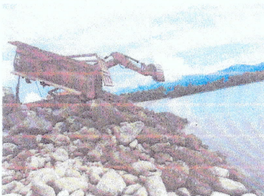
Picture Nos. 36 & 37: Left- Dumping of Armor rocks at the east portion of Phase 2; and Right – Placing the core and armor rocks (taken Aug. 4, 2022 PM)
