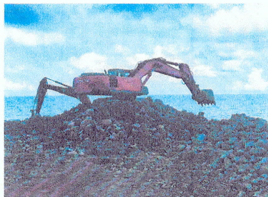
Picture Nos. 29-30, Left - core rock placement as of July 23, 2022 and right, Causeway image at 410m length as of July 25, 2022
