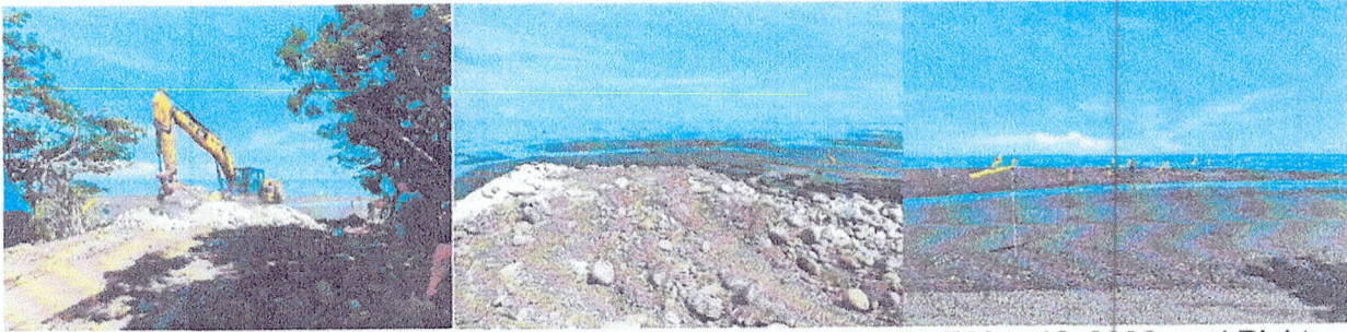
Picture Nos. 11-13: Left- Causeway advancing along the beach of May 12, 2022, and Right- Dumped and spread materials at the edge of the Causeway showing the guide stakes along the beach for dumping of core and armor rocks as of May 14, 2022.
