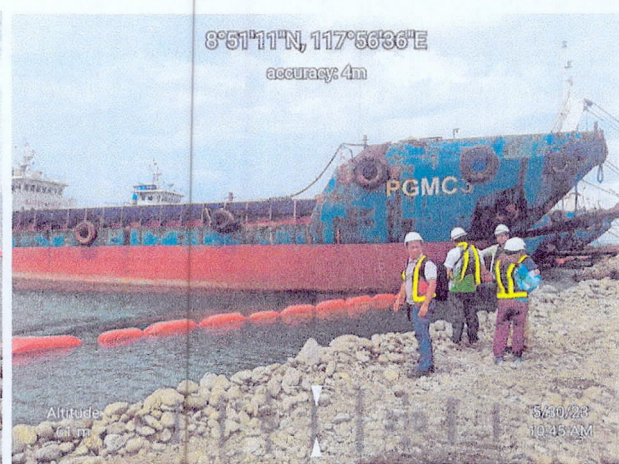
Installed silt curtain to avoid sediment dispersal
