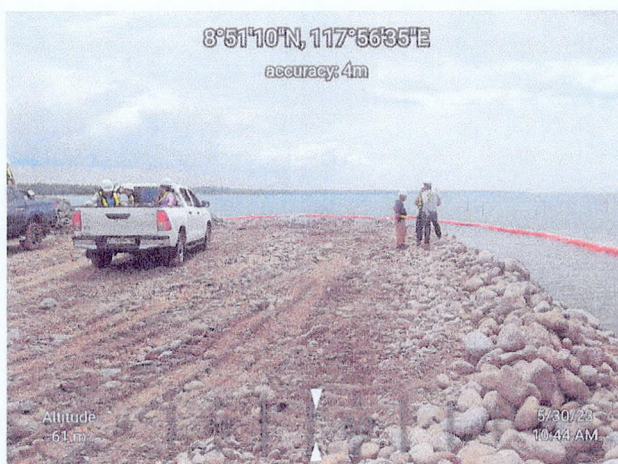
Installed silt curtain to avoid sediment dispersal
