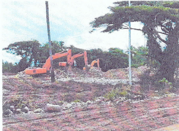
Picture No. 31: Three (3) backhoe excavators doing sorting of Core and Armor Rocks
