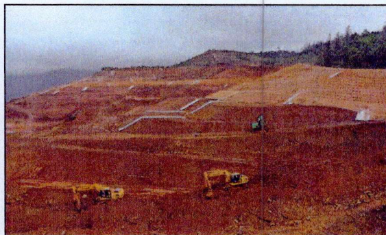
Bench/Slope Correction Works
