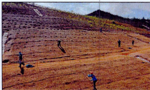
Installation of Coco coir Mats on benches
