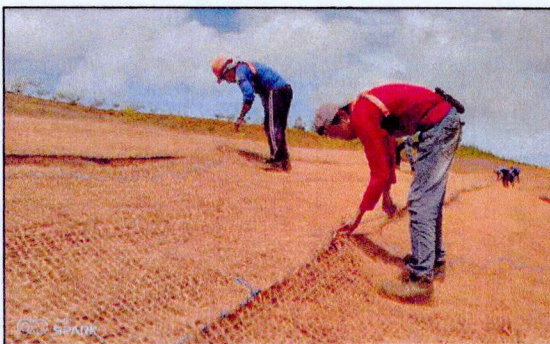
Installation of Coco coir Mats on benches
