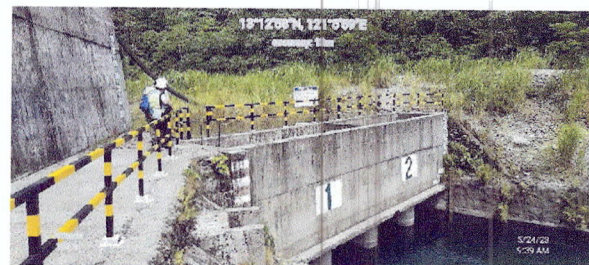
Tail Race where the water from the palnt is being discharged
