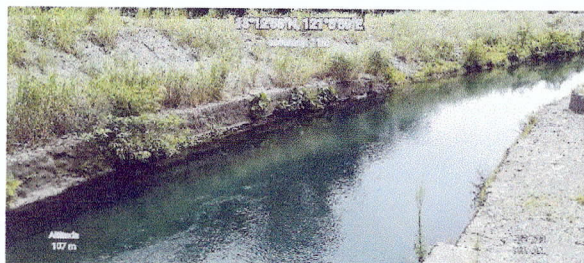
Tail Race where the water from the palnt is being discharged
