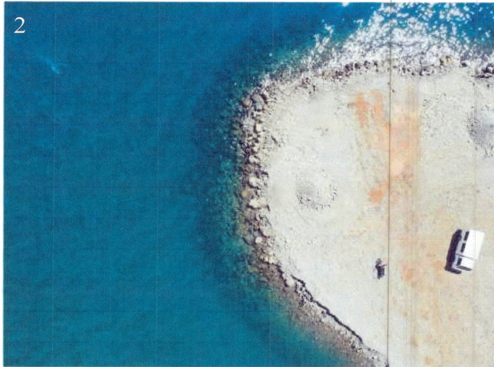
Figure 10. Drone shot over causeway.
