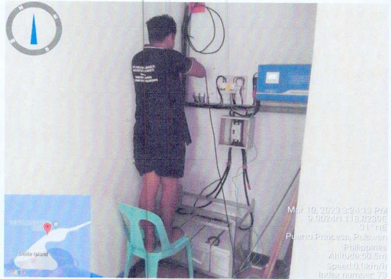
Photos during the installation of solar charger controller and re-wiring of electrical system
