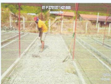
HAULING AND BACK FILLING OF GRAVEL AND SAND ALONG THE PATHWAY OF SEEDLING BED
