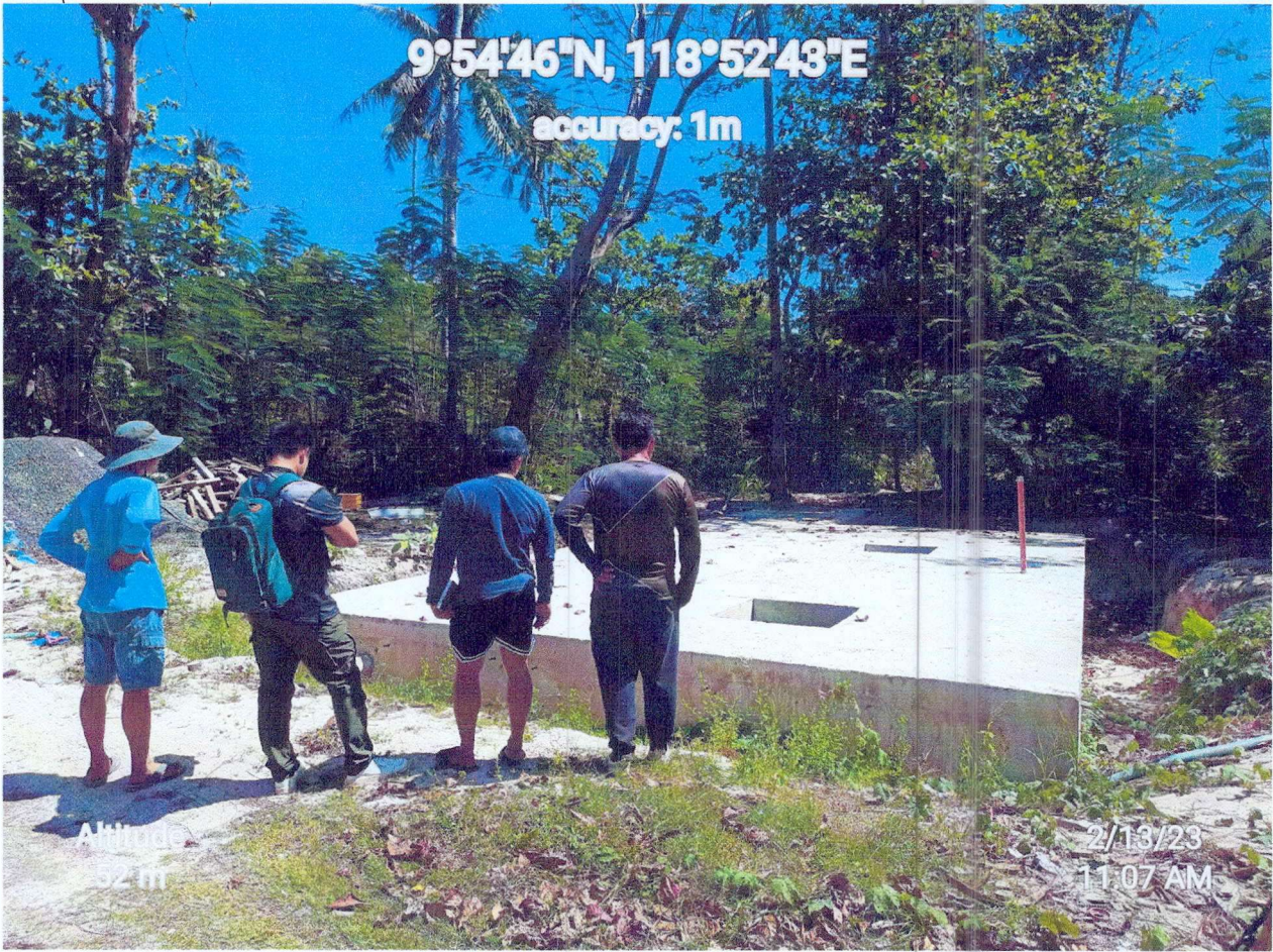
Figure 3 Photo shows the newly constructed STP holding Tank
