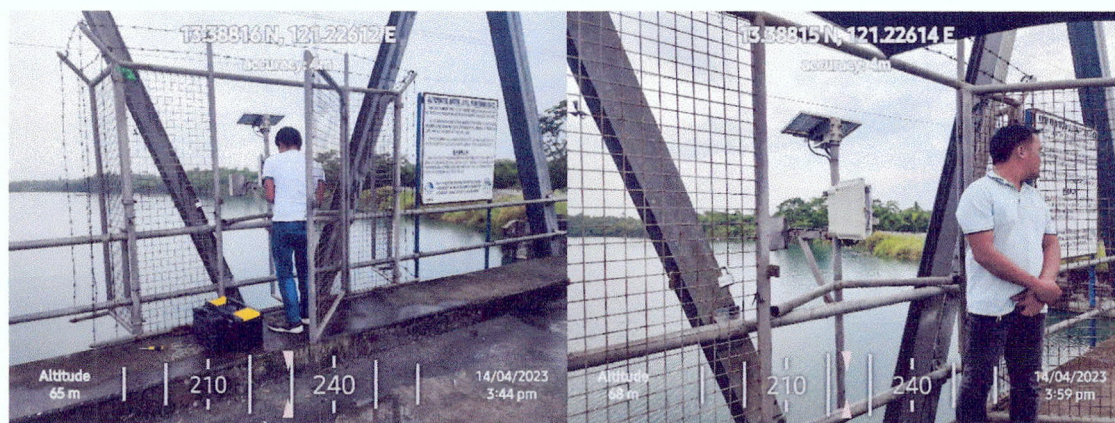
Figure 2. Installation of new solar panel and solar charge controller in Abaton AWLS station
