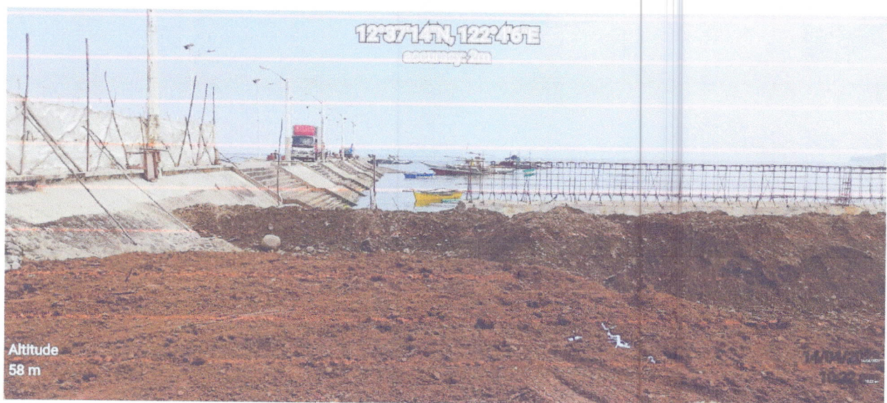
Continuous filling up/spreading of earth soil to the embankment
